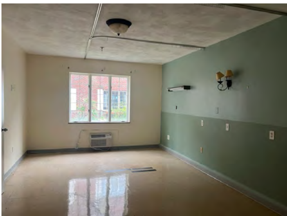
Interior – Existing Condition
