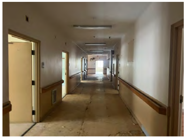
Interior – Existing Condition
