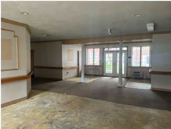
Interior – Existing Condition
