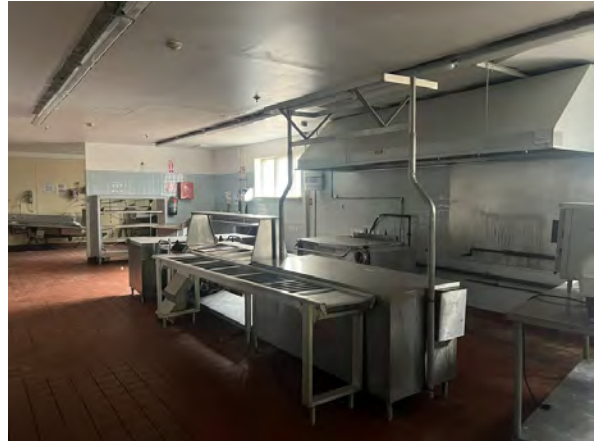
Interior – Existing Condition
