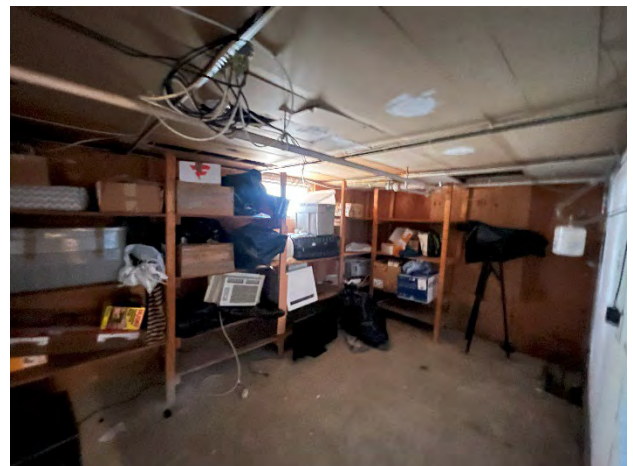
Unfinished basement, storage area
