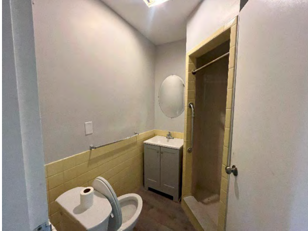
Second floor, bathroom 1
