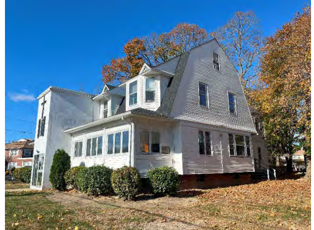
Front/side view of the subject from SE corner
