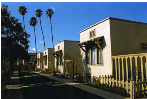
Hollywood Bungalow Courts, Los Angeles, California (1921-1925). Rehabilitated as housing for special-needs and low-income residents. Photograph: NPS Files.
