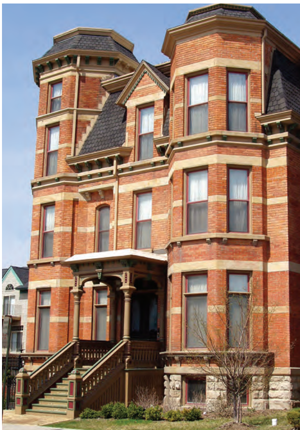
John Harvey House, Detroit, Michigan (1875). (opposite) Before rehabilitation; (above) After rehabilitation as a bed and breakfast. Courtesy: Marilyn Nash-Yazbeck. Photograph: Steven C. Flum, Inc.
