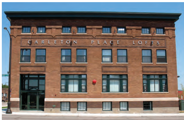
Carleton Place (historic name: Simmons Manufacturing Company), St. Paul, Minnesota (1909). Before and after rehabilitation for residential use. Courtesy Hess, Roise and Company.
