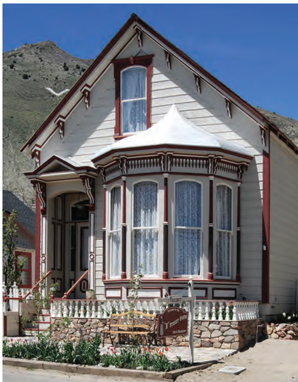
58 B Street, Virginia City, Nevada (1875). Rehabilitated as a bed and breakfast. Courtesy Chris Eichin.
