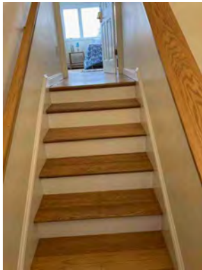
Stairs to third floor
