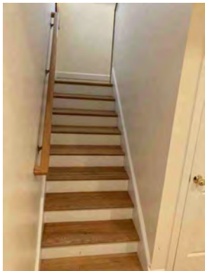
Stairs to second floor
