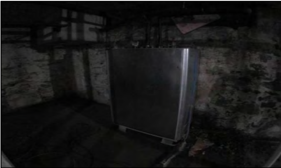
49 Elm St oil tank
