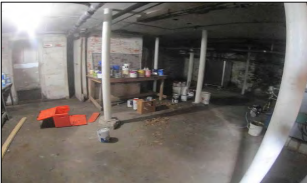
49 Elm St BASEMENT
