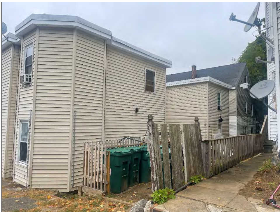
Subject East Side Exterior
