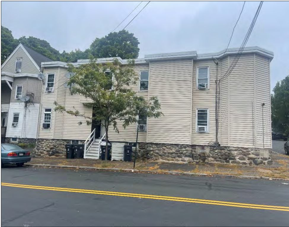
Subject West Side Exterior
