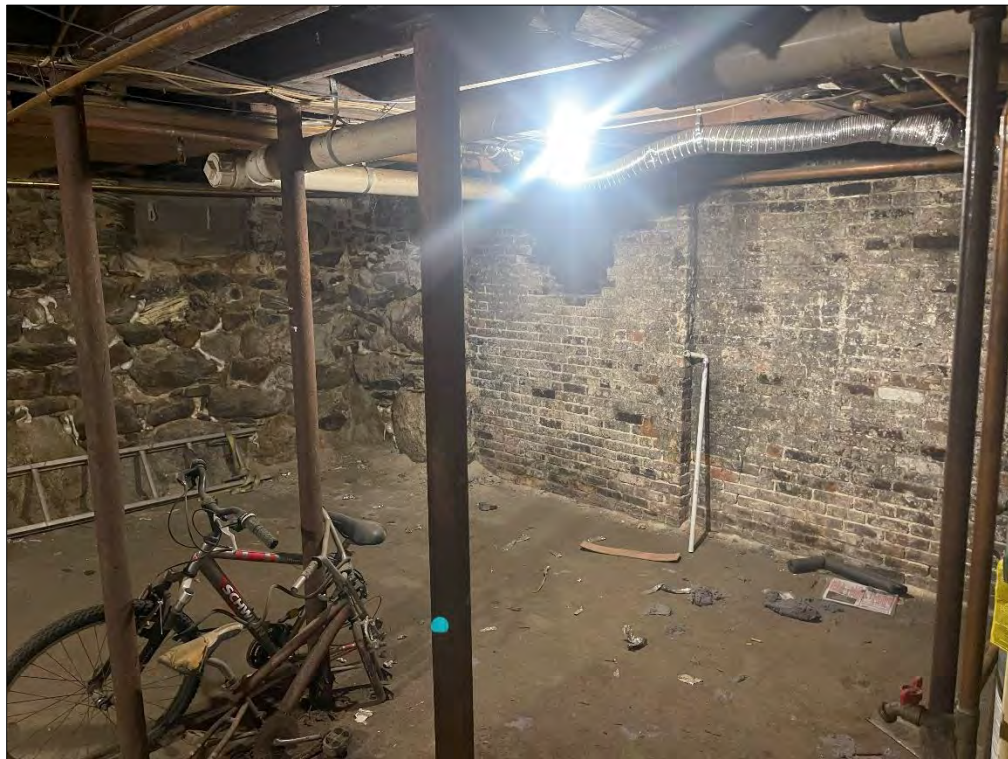
Typical Basement Interior
