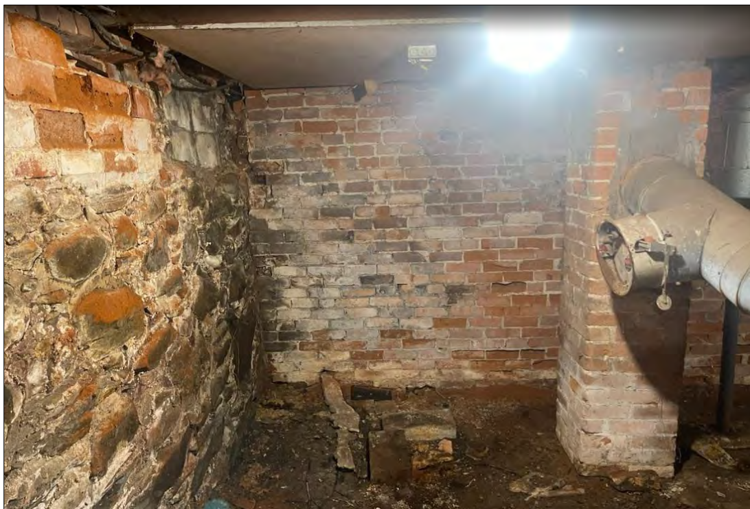
Typical Basement Interior
