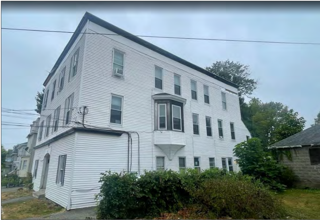
Subject East Side Exterior
