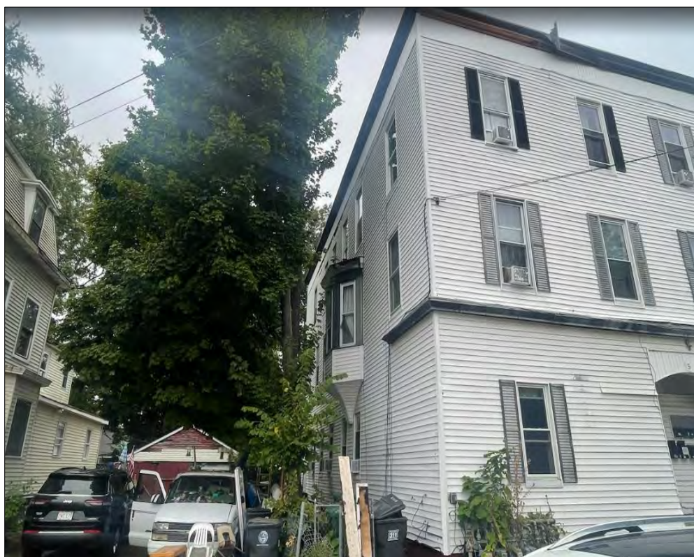
Subject West Side Exterior
