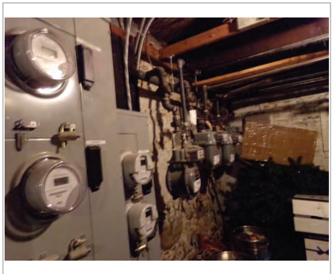
LOWER LEVEL - UNFINISHED BASEMENT
