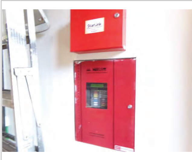
INTERIOR - COMMON AREA
