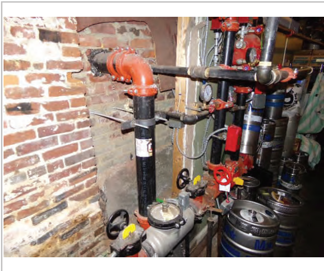
LOWER LEVEL - UNFINISHED BASEMENT
