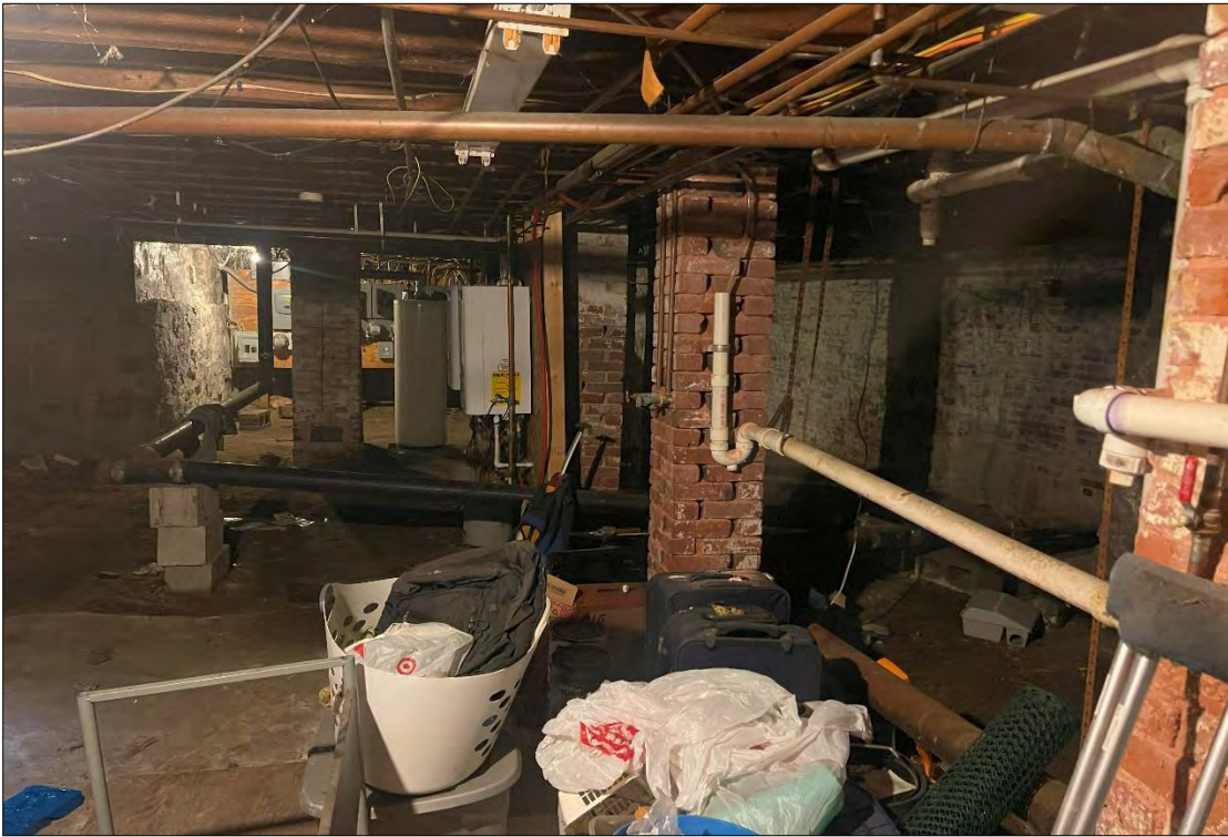
Typical Basement Interior
