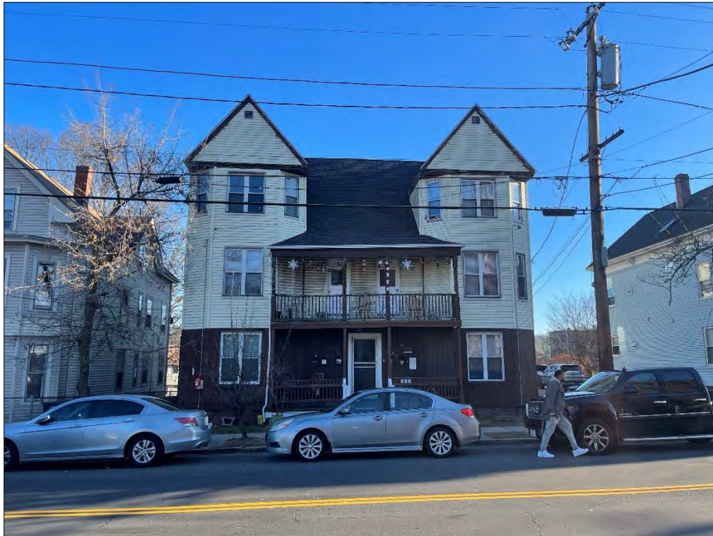
Subject North Side Exterior
