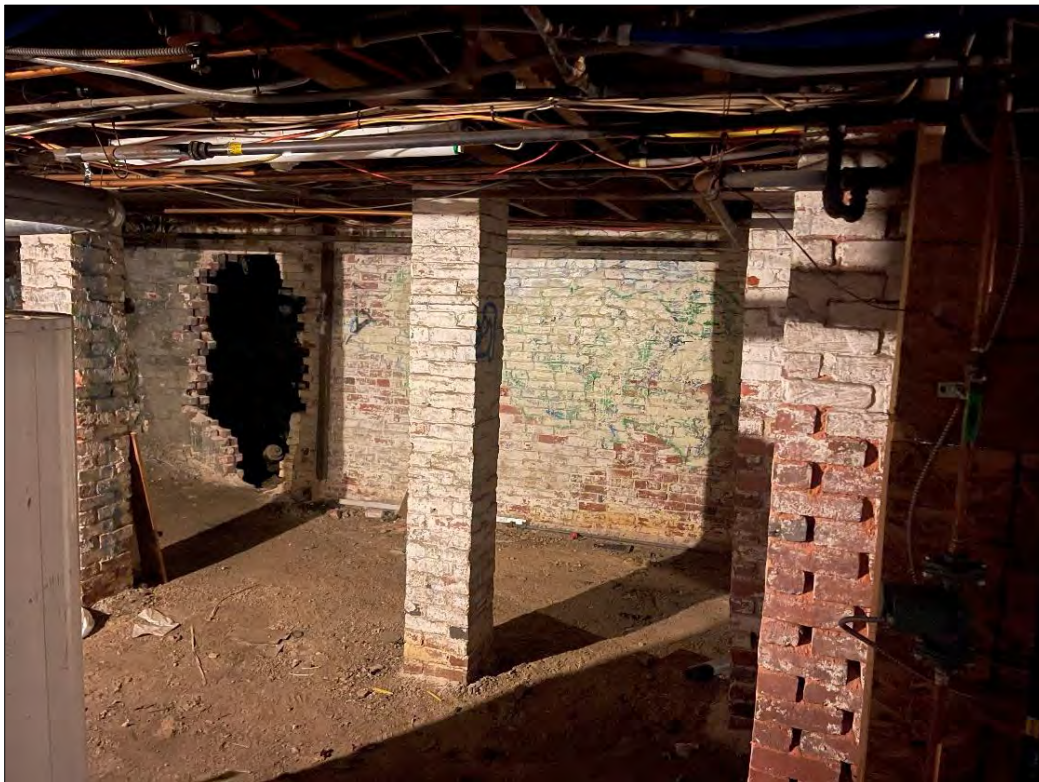
Typical Basement Interior
